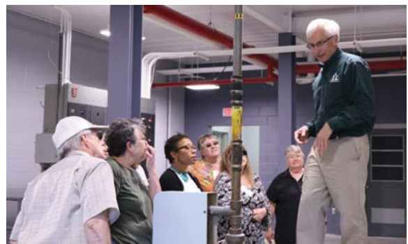
Richard "Dick" Lorenz explains how the Water Treatment Plant works to a tour group.
